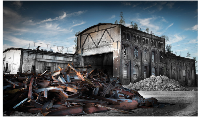
Alphonse Colling, Destruction Esch Terres rouges
