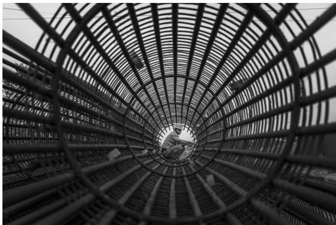
The daily work of pipe fitter - Baozhong Yang , China
